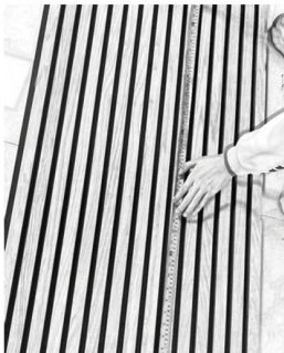
② Measure the wooden slat acoustic panel
